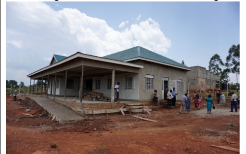
Much progress at the new medical clinic.
